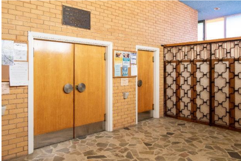
Narthex showing doors through to nave with 'crying room' on right Source: DEW Files 28 January 2021
