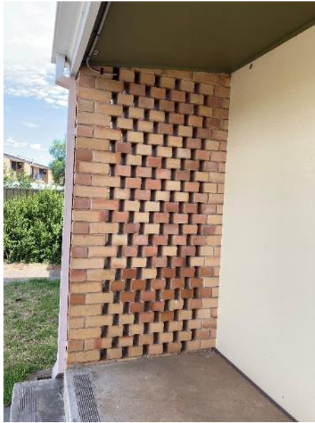
Hit-and-miss cream brick screen adjacent to porch at northern end of church Source: DEW Files 28 January 2021
