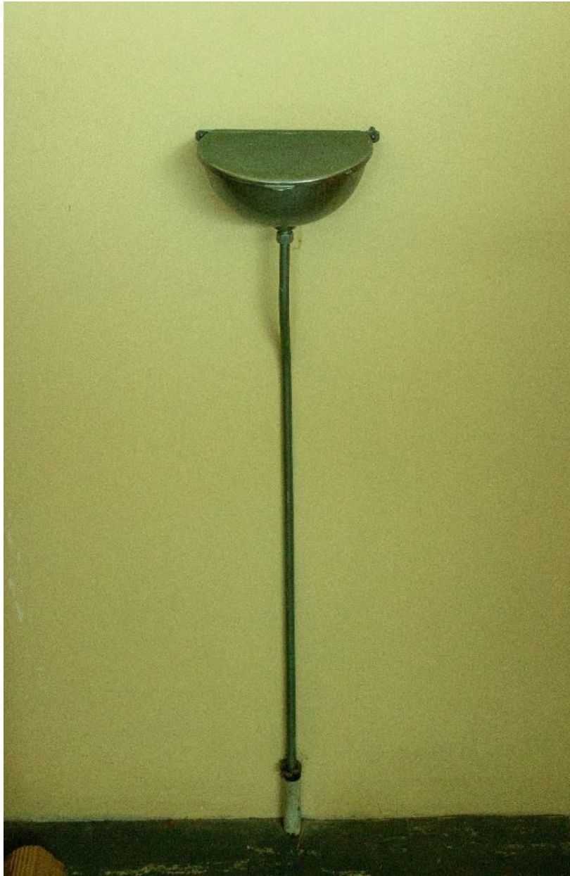
Sacrarium (sanctified drain) in sacristy
