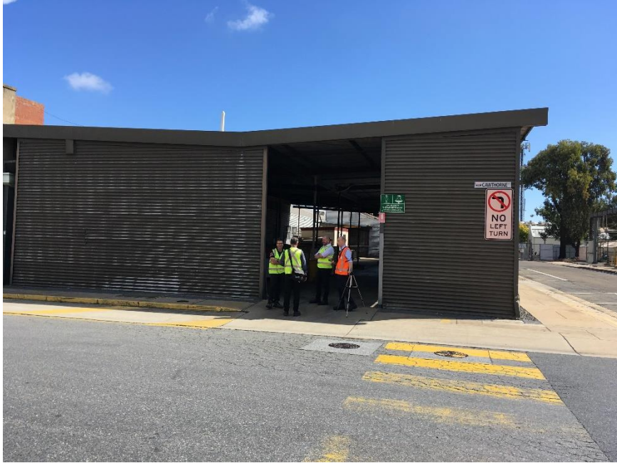
Corner of Cawthorne and Winwood Street showing the shed.
