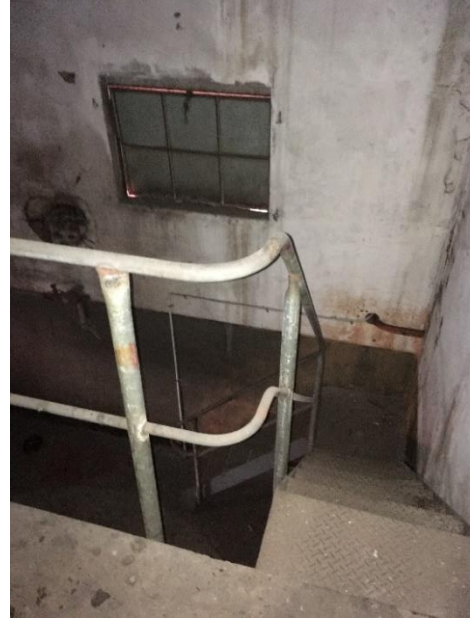
Inside the Brewhouse Tower, showing the space as it remains after decommissioning.
