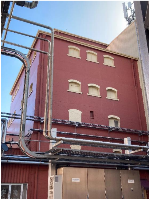
Walkerville Brewhouse Tower showing eastern and southern elevations.
