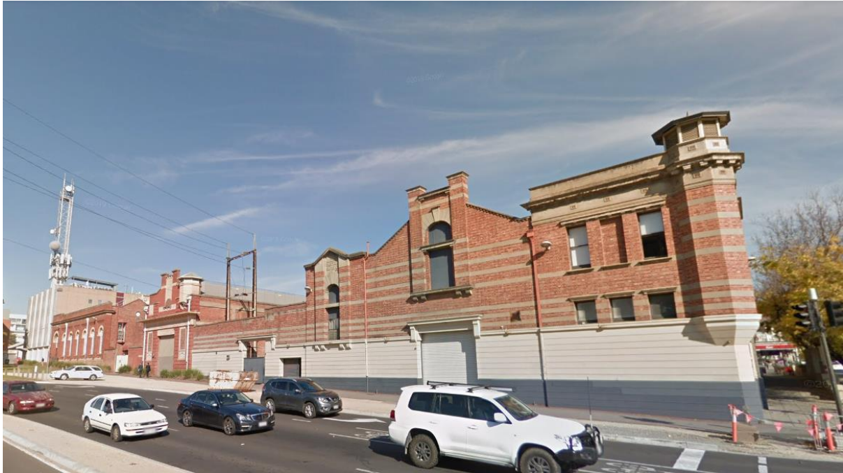
View of East Terrace showing Tandanya (former Adelaide Electric Supply Company Power Station) (SHP 10984) (right), Former Adelaide Electric Supply Company Converter Station (SHP 10985) (mid) and Former Municipal Tramways Trust (MTT) No.1 Converter Station (SHP 10986) (left).
