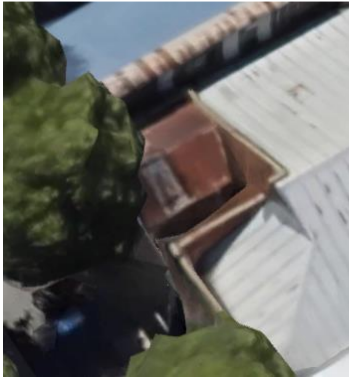
View of the transformer showing the structure behind the fence.
