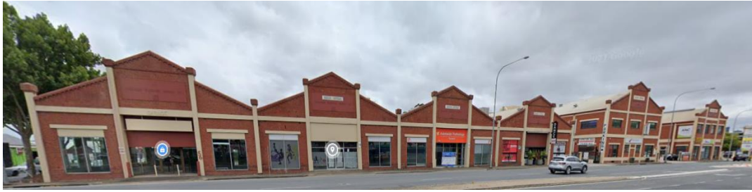
Former Adelaide Electric Supply Co Ltd - Four former garages and two double storey office/workshop buildings (SHP 26308)
