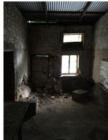
Interior images of the Outbuilding
