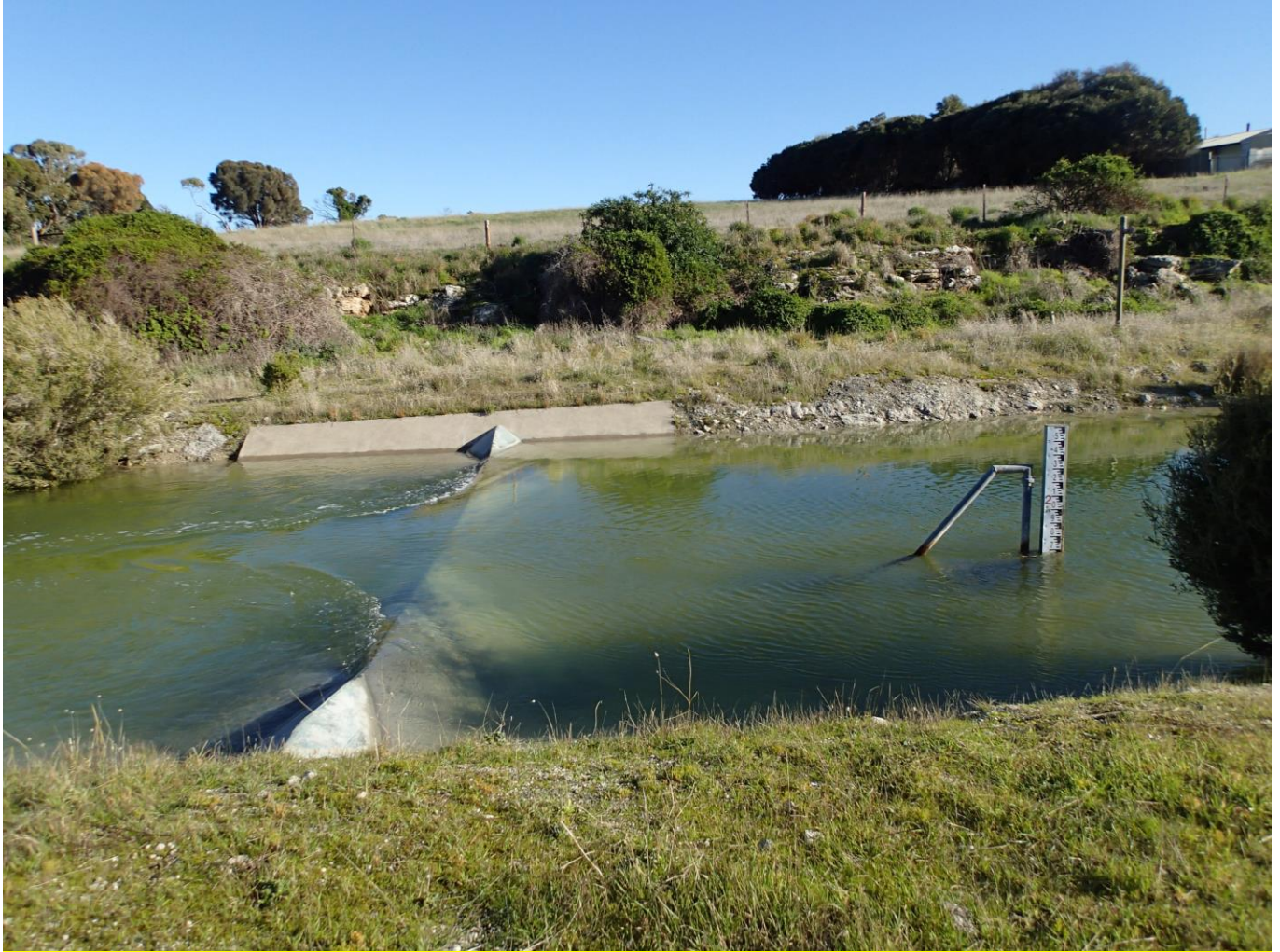
Figure 1: Salt Creek in the States South East. All freshwater released from Morella Wetland through Salt Creek and into the Coorong's South Lagoon flows over the pictured concrete flow gauge (or wedge). On the downstream side of the flow gauge, a small pipe fills a composite sampler nearby (not pictured).
