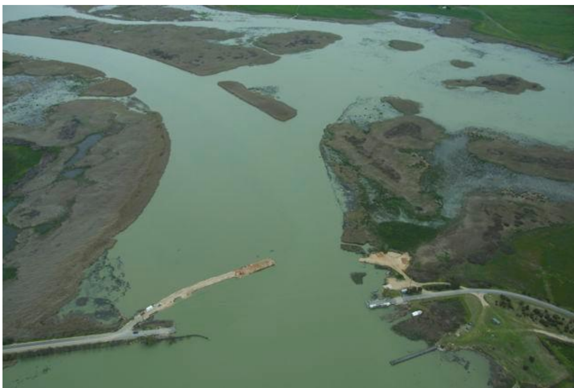
Figure 10: Narrung causeway and partial remains of the temporary bund, August 2010
