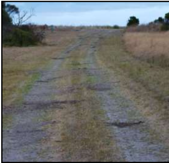
Figure 8: Rabbit damage in main track
