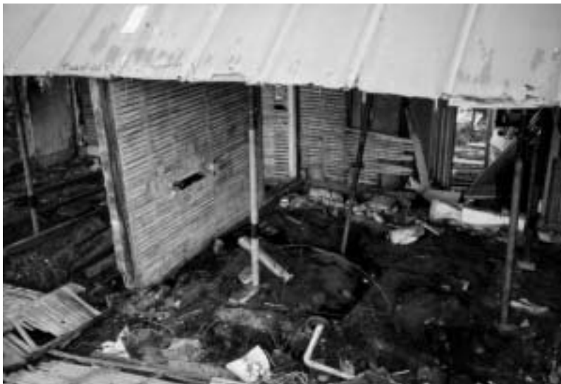
below: Bedroom of the original cottage before and after restoration.
