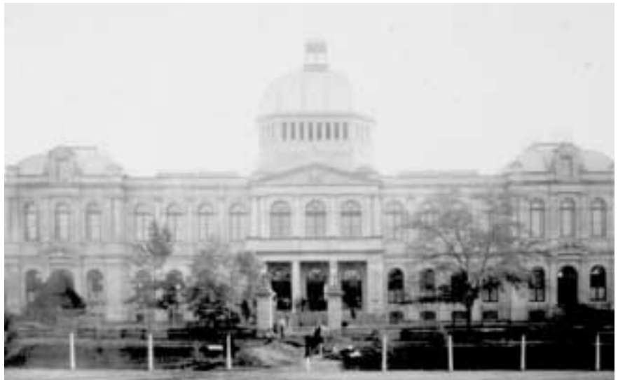
Jubilee Exhibition Building erected 1887. Demolished 1963
