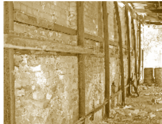
Three original Down-Draught Brick Kilns and Chimney, Krieg's (previously Nuriootpa) Brickyard, Murray Street, Nuriootpa.
