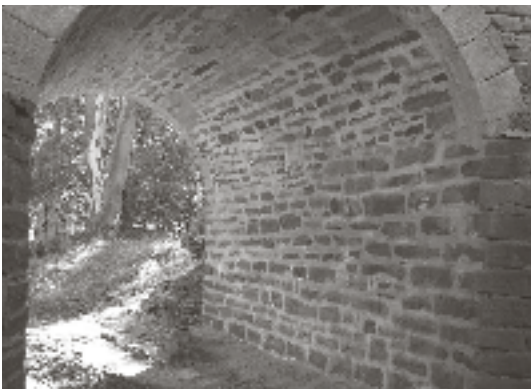
Ross Creek Bridge, Kapunda, after repair
