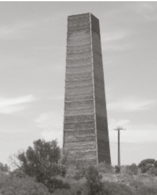
Hughes Chimney Stack, Wallaroo
