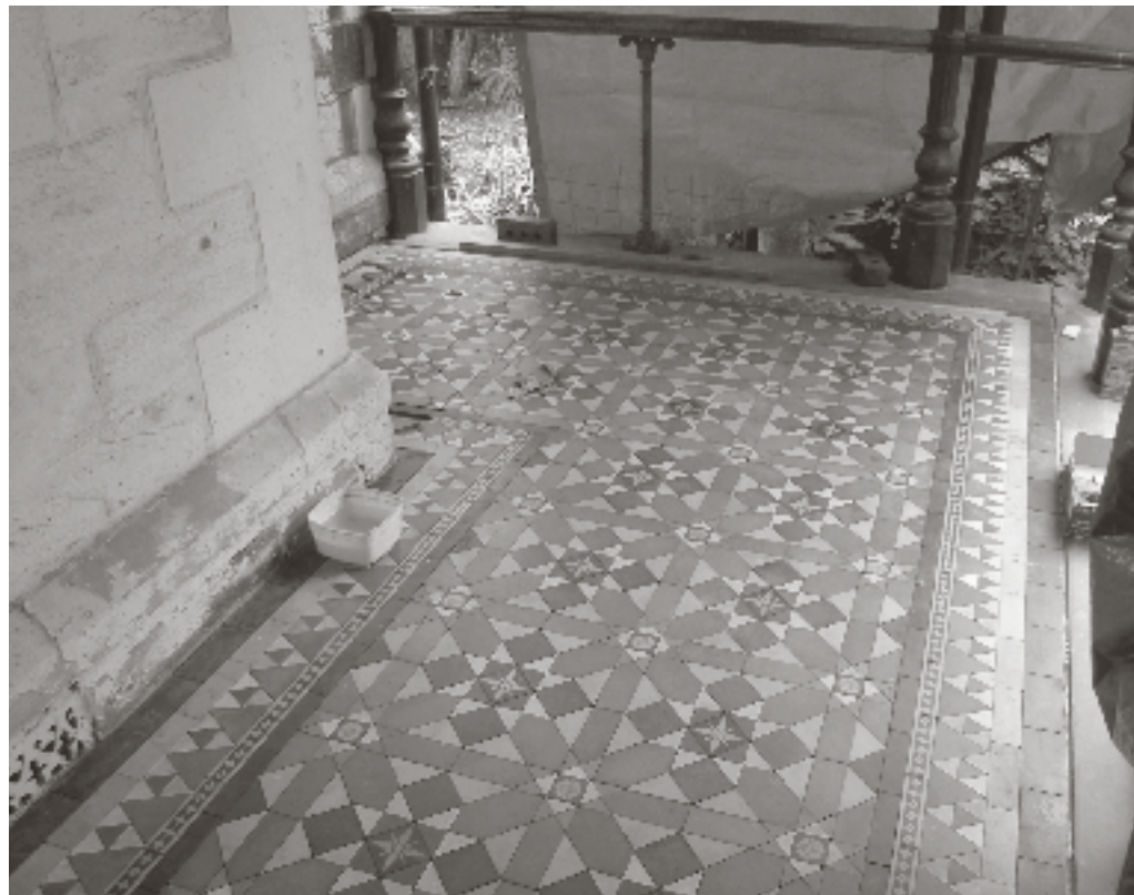
Korra Weera, Marden, veranda tiles after repair
