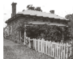
Former Powder Magazine Keeper's Residence, Adelaide.
