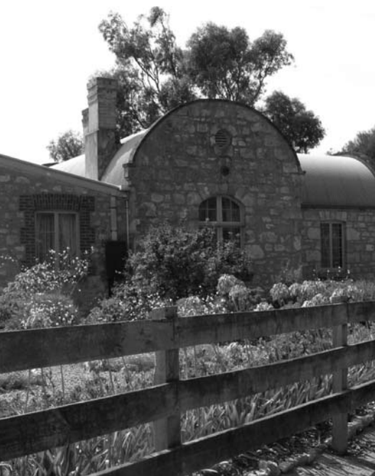
Former Railway Superintendent's House, Goolwa
