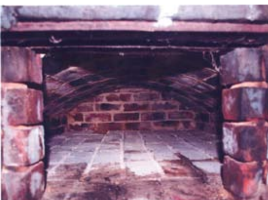
Oven after conservation, Keil House smokehouse
