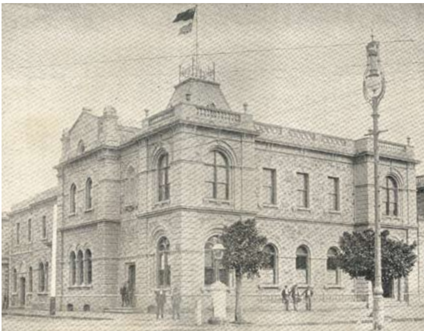
The Port Adelaide Institute as it appeared in Meleng's 1902 book (facing p13).
