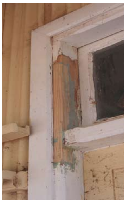
Repaired door frame, Morgan Railway Station (2007)
