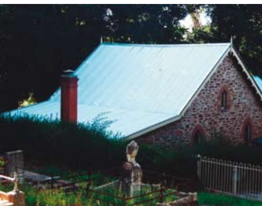
Salem Church after re-roofing (2007)
