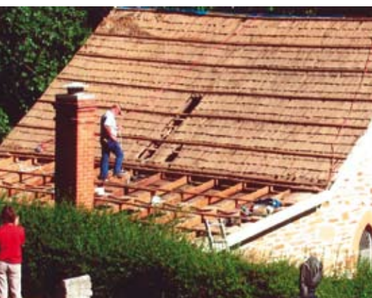
Timber shingle roof exposed during re-roofing (2007)
