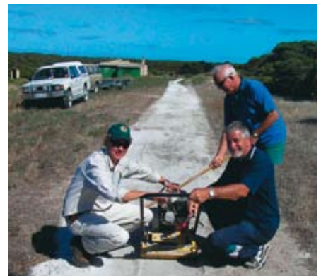
Trail upgrade by Friends of Innes National Park
