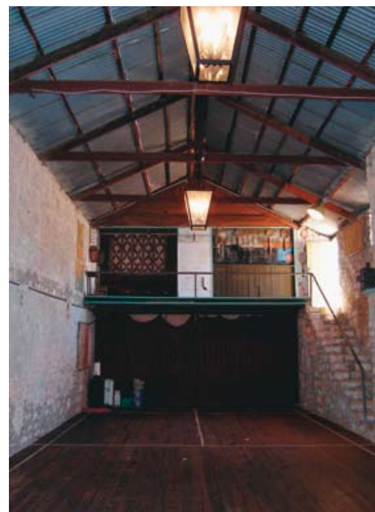
Woolshed turned badminton court, Nor'West Bend Station
