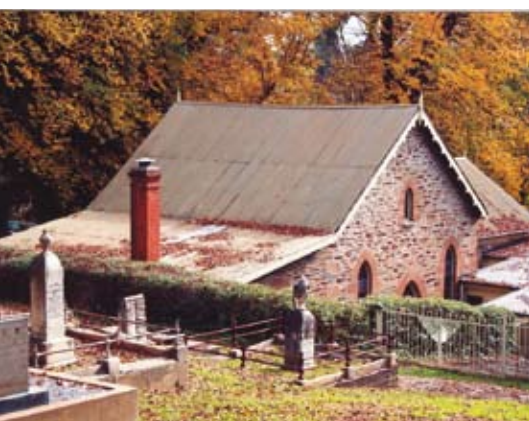
Salem Church before re-roofing
