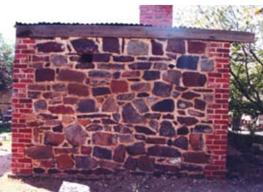
Rebuilt wall of smokehouse
