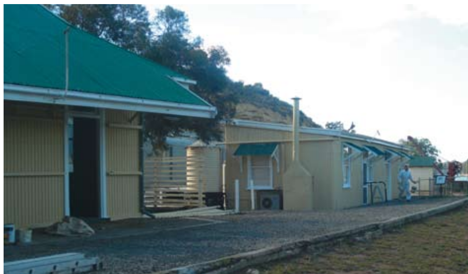
Structurally sound and newly painted, the Morgan Railway Station Ticket Office and Refreshment Rooms (2007)
