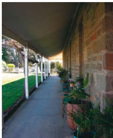
The homestead is constructed from bluestone sourced from the property, Rhine Park (2007)
