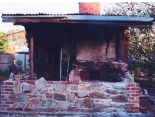
Keil House smokehouse during restoration work
