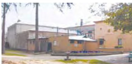
Mt Gambier City Hall before redevelopment.
