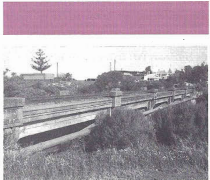
Hindmarsh River Bridge near Victor Harbor is Australia's first reinforced concrete girder bridge. The bridge was built between 1905-1907 and reflects the prosperity of the Victor Harbor region in the early twentieth century.
