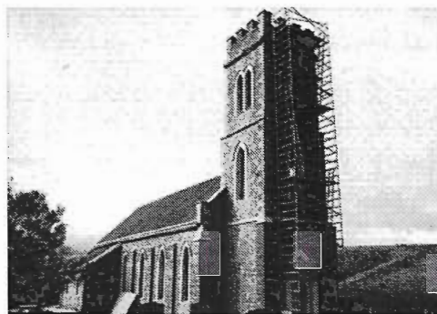
St Phillip & St James Church in the process of restoration.
