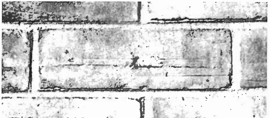
Above: Hack marks on a hand-made brick.
