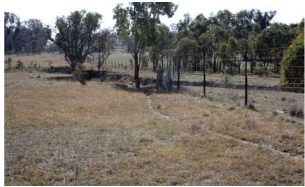
3 strand plain wire fence affixed to the top of a stock-proof fence to exclude kangaroos Photo: Graham Hodge
