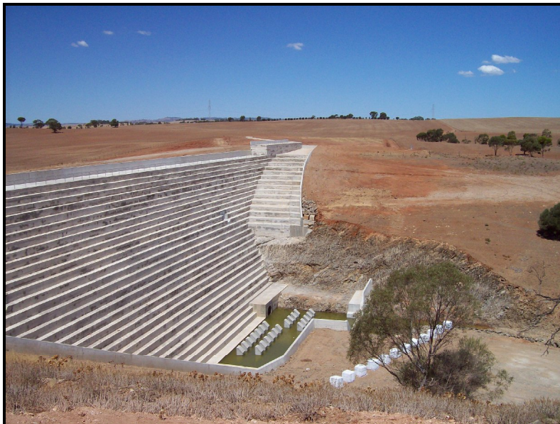
Flood Mitigation Dam – Gawler River
