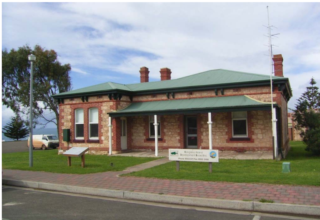
View of former Police Station from Kingscote Terrace
