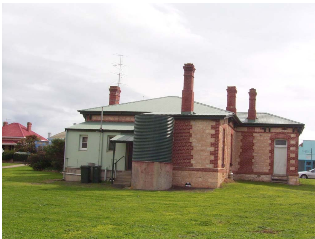
Rear view of former Police Station
