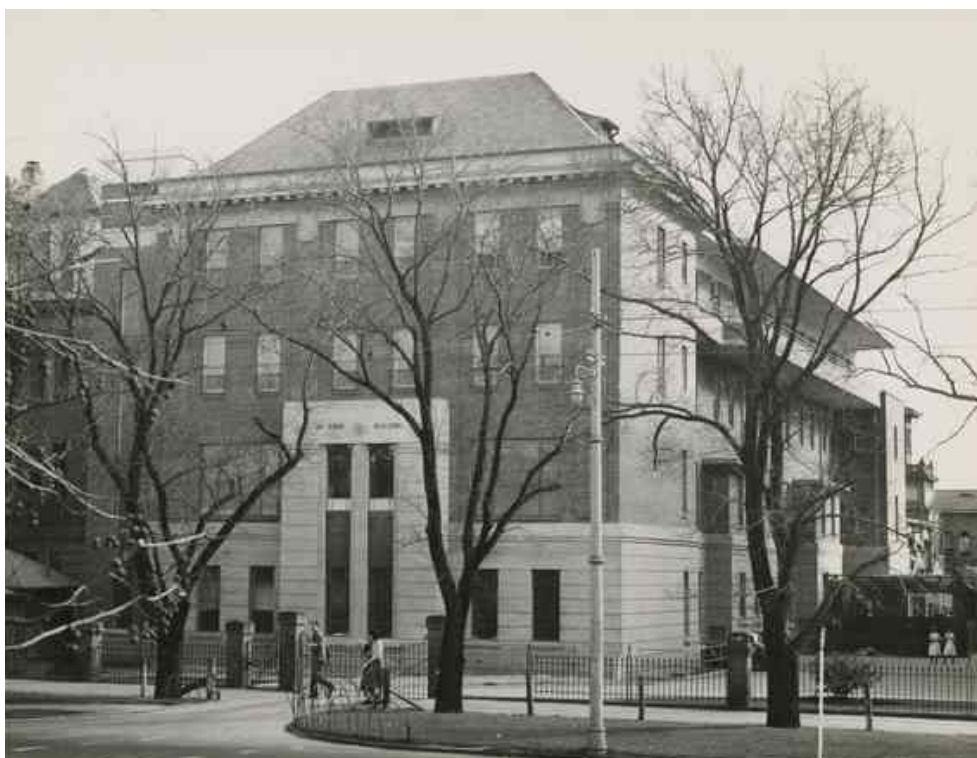
McEwin building soon after opening in 1946 (Source: SLSA B14019)
