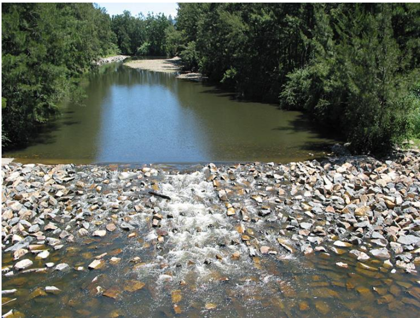
Figure 18. A full-width rock-ramp fishway.
