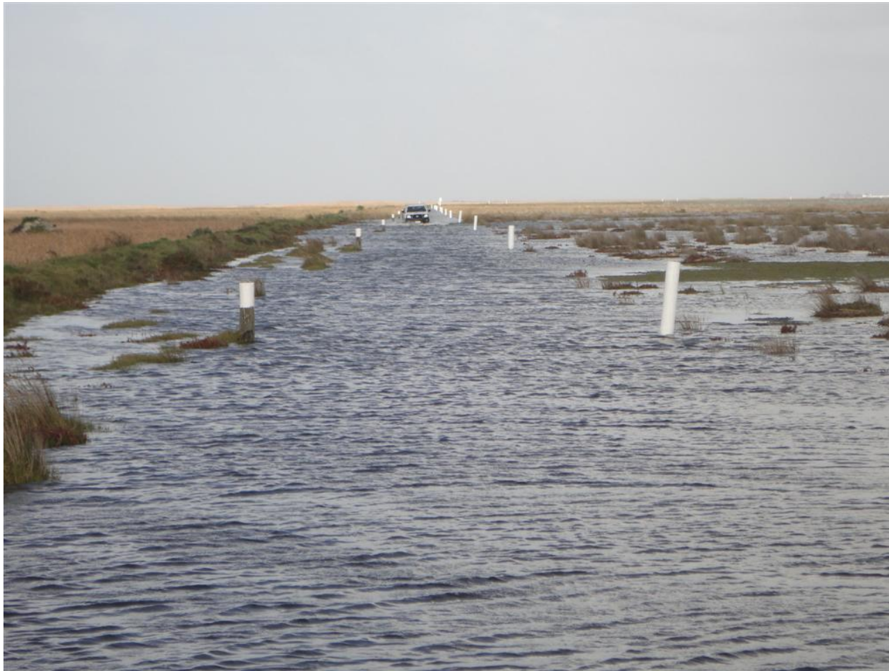
Figure 30: Reverse Flow at the spillway site 17 August 2011
