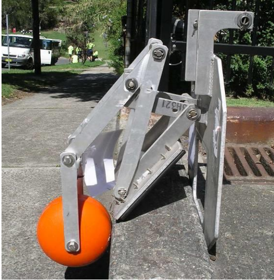
Figure 20. Float-operated gate used for fish passage on tidal floodgates in NSW.
