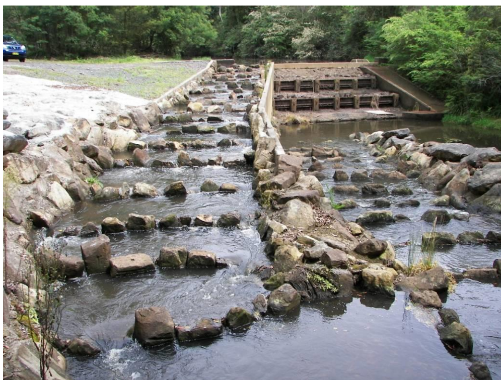
Figure 19. A partial-width rock-ramp fishway.
