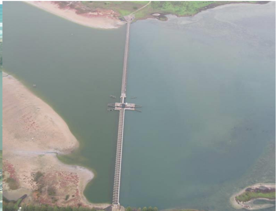
Figure 23. Aerial of Goolwa Barrage
