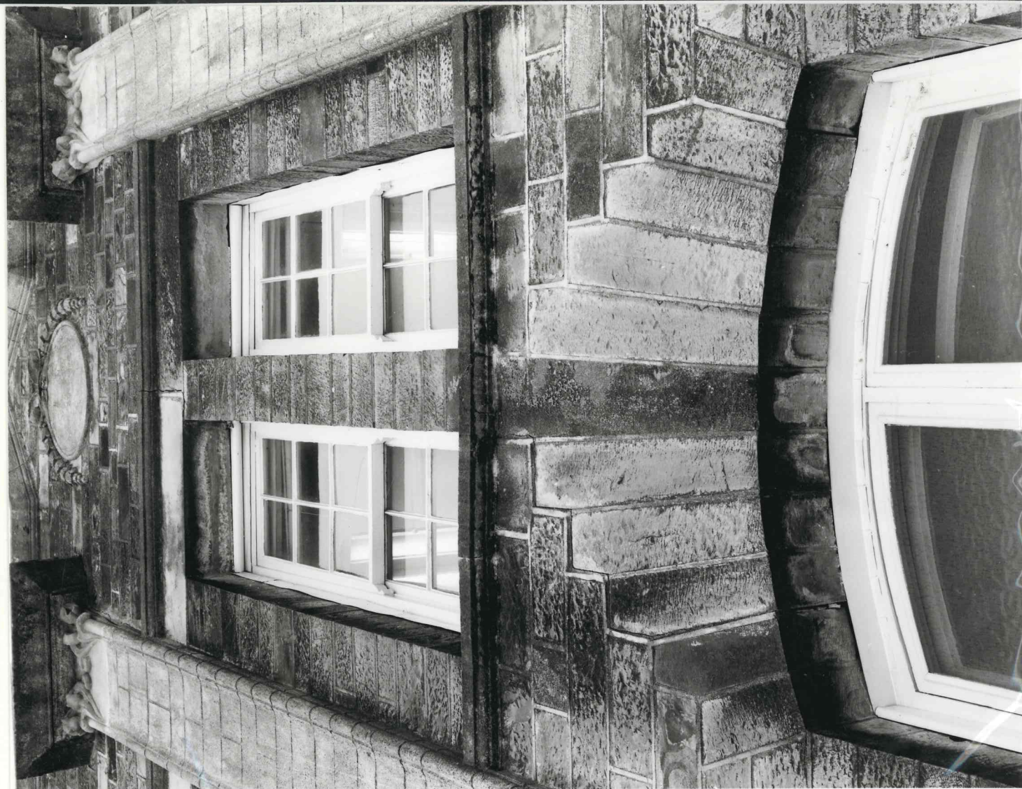
FILM 31 ELECTRICITY TRUST BUILDING, DETAIL OF NO 3 MAIN NORTH RD FACADE
