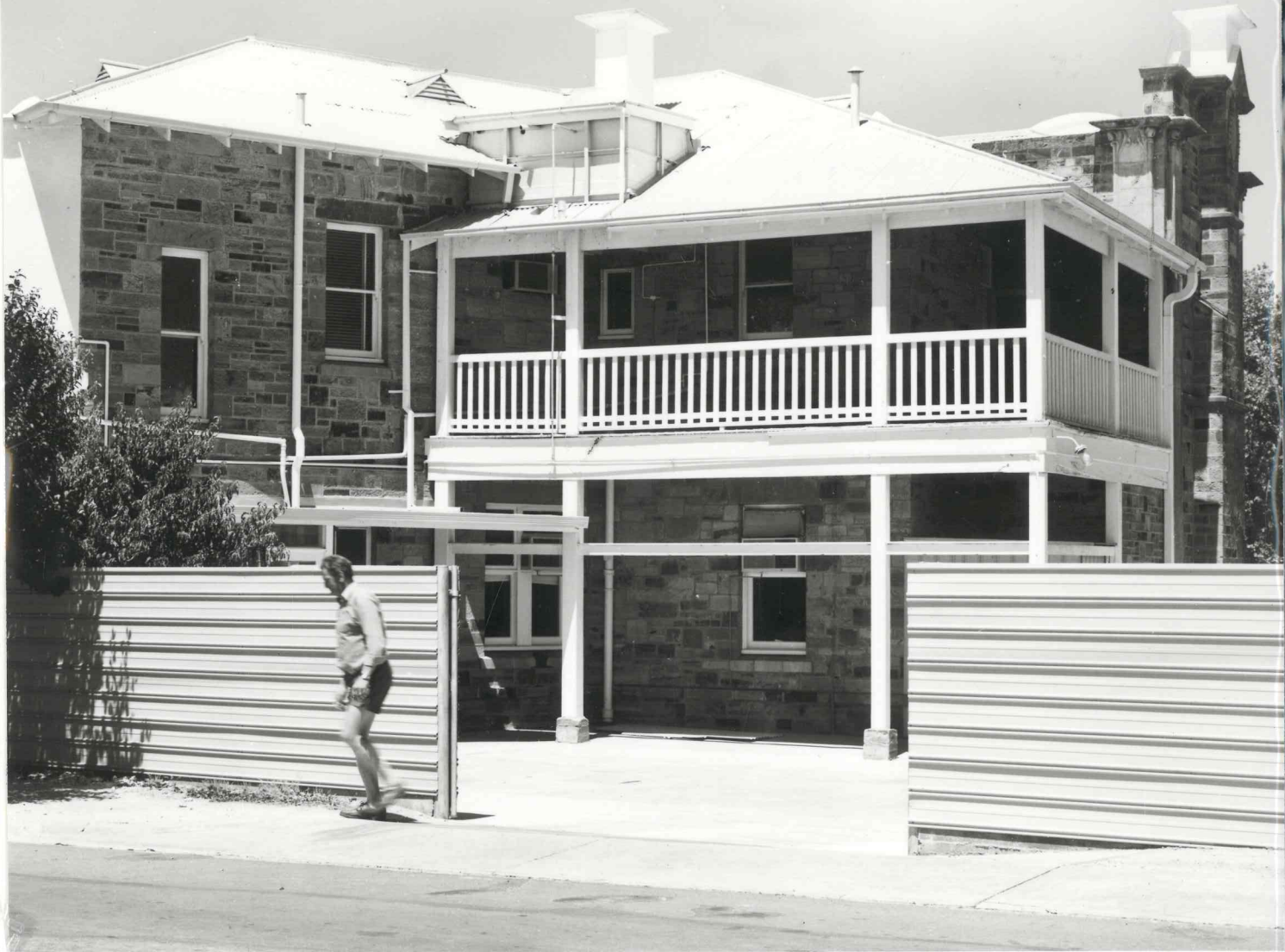
FILM 31 ELECTRICITY TRUST BUILDING, FROM NO 5 OLD NORTH ROAD.
