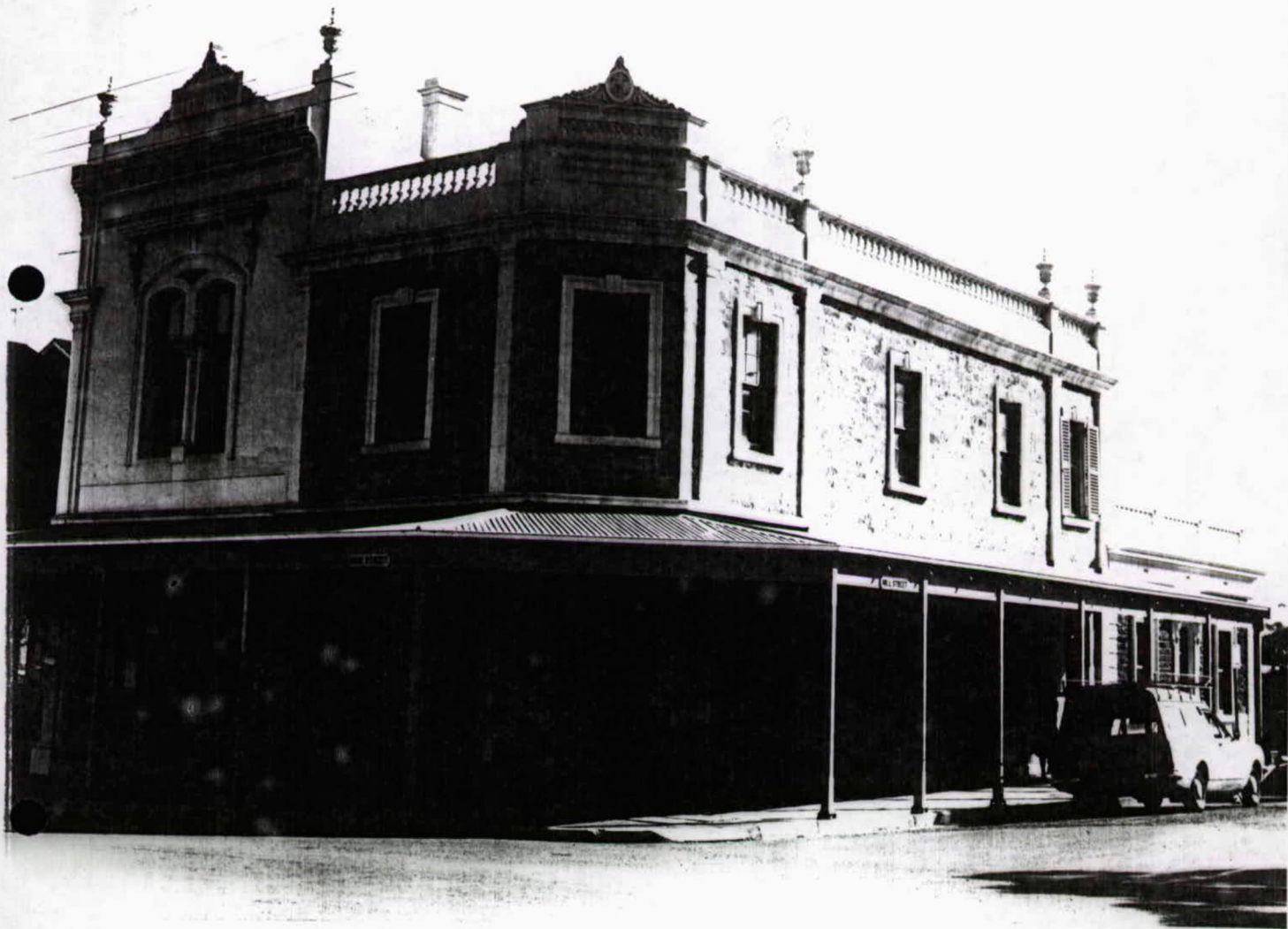
Thomson Building, Corner Main + Hill Sts, Kapunda.
