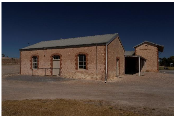
South-eastern facade of Pavilion and Grandstand.
