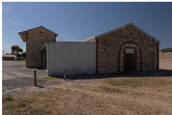
North-western facade of Pavilion and Grandstand with closed in corrugated verandah.
