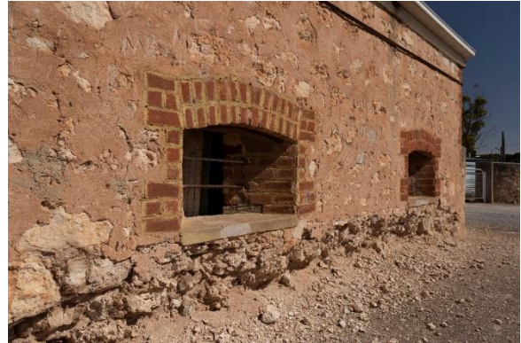
South-eastern façade of Ticket Office with window detail.
