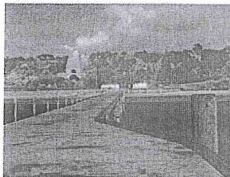
Jetty and Lime Kiln, Wool Bay (Photo: R Ashworth 2005)
