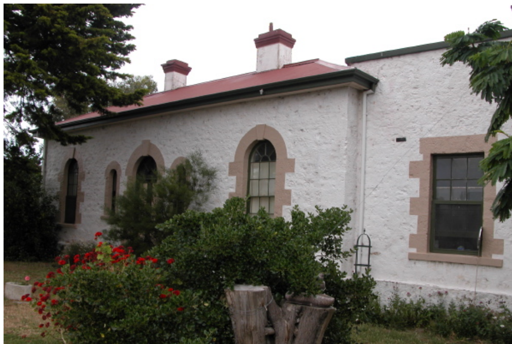
Police Station, front wall from NE
