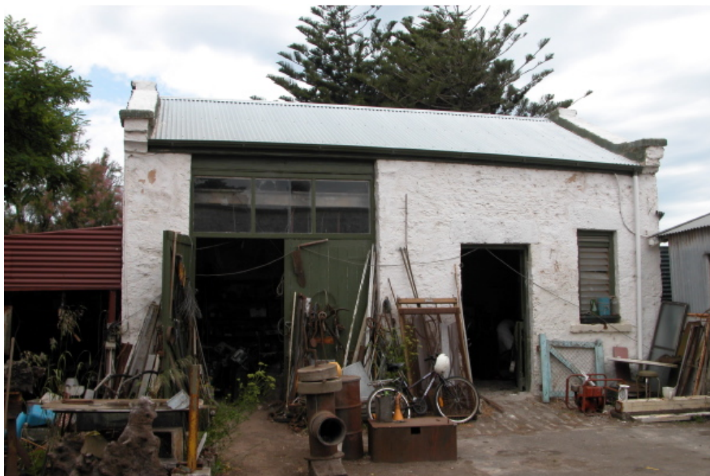
Stables at rear of Police Station
