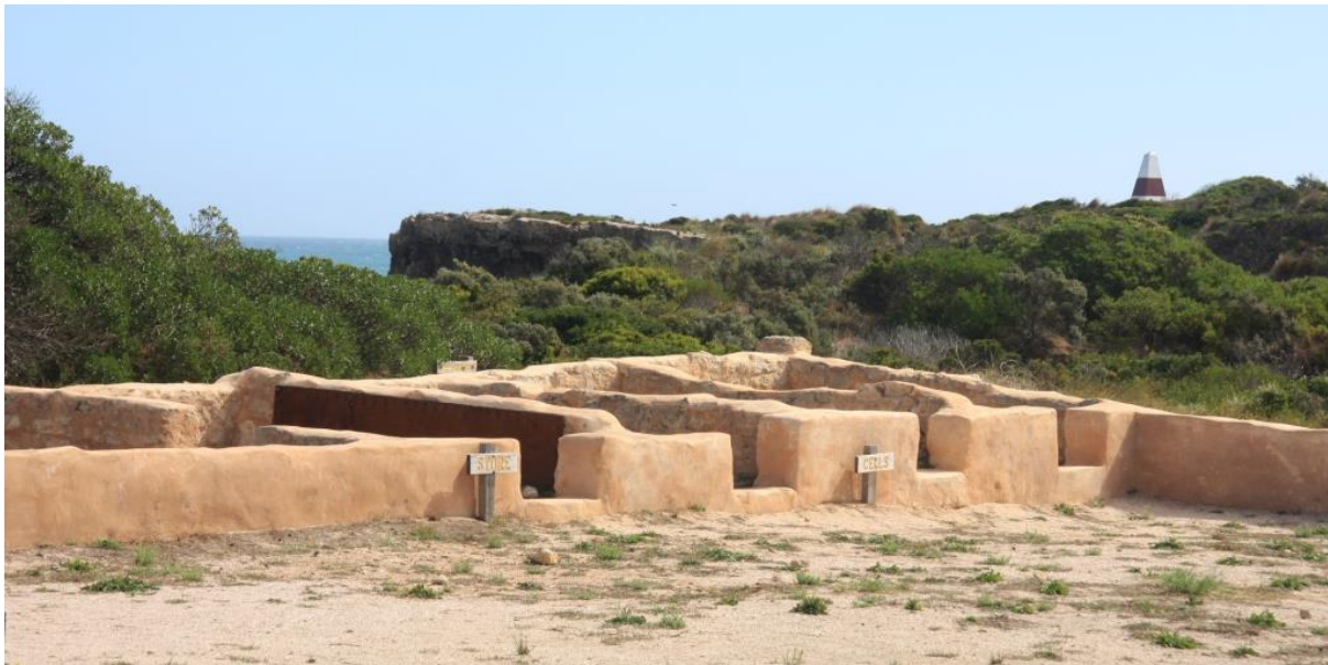
The Gaol Ruins, c.2012 after the remaining walls were stabilised and partially rebuilt in 1995 to assist in interpreting the site. Note the Cape Dombey Obelisk in the background.
