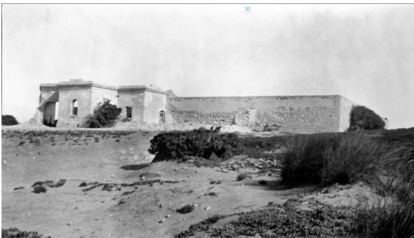
The Gaol Ruins in 1924. A portion of the perimeter walls are still standing, however, the chimneys, roof and wall (mid left) appear to have fallen in or been removed.
