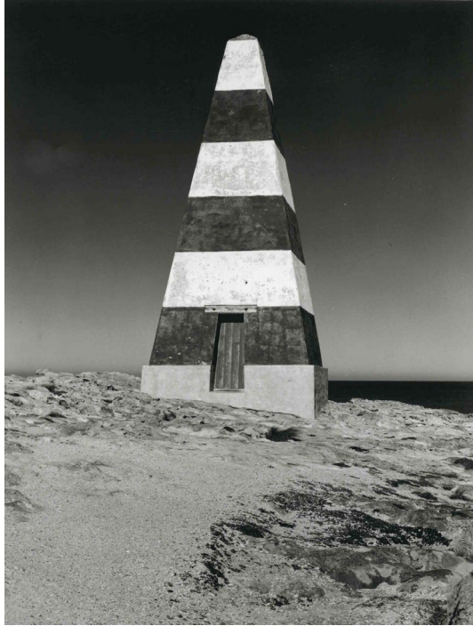
The Obelisk in 1979, the year before it was listed as a State Heritage Place. Note the wooden lintel and door.
