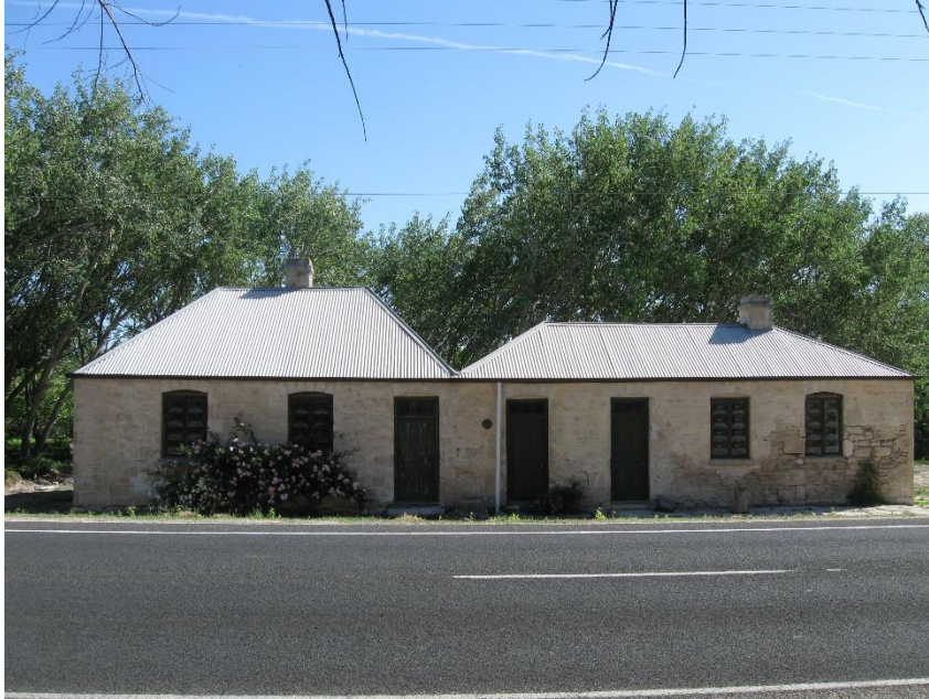
The Bush Inn following conservation works, including reroofing, 2009.
