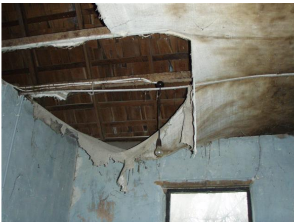
Interior of Bush Inn prior to conservation work showing torn calico ceiling, c.2008.
