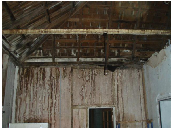
Interior of Bush Inn prior to conservation work showing timber shingles, c.2008.
