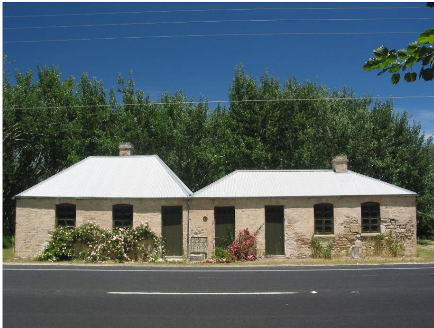
The Bush Inn following conservation works, including repointing, 2003.
