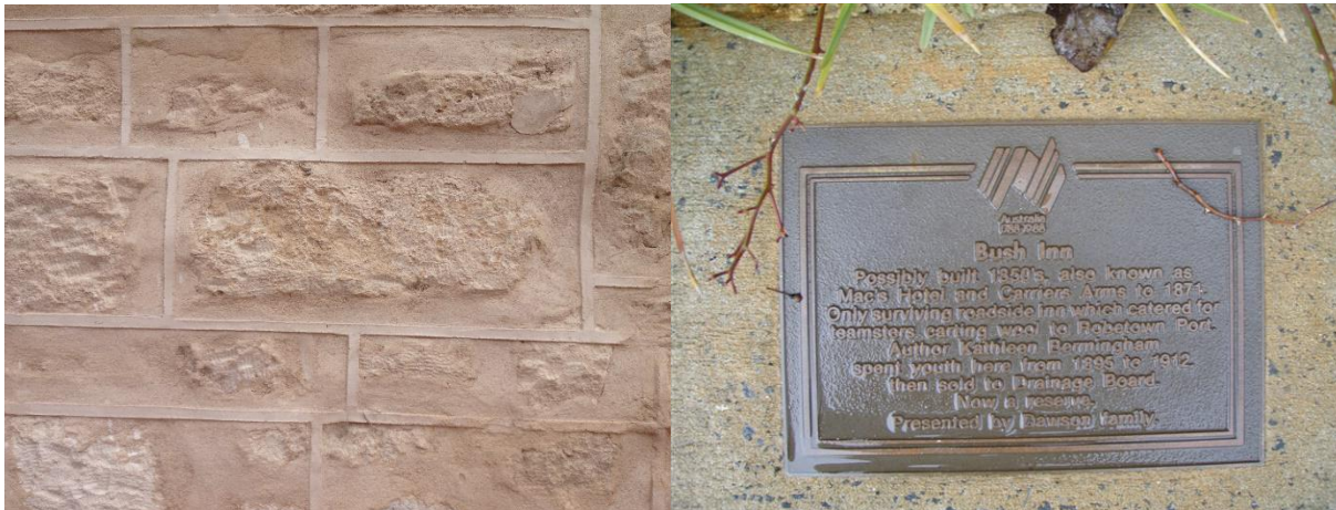
Repointing work, c.2013.
