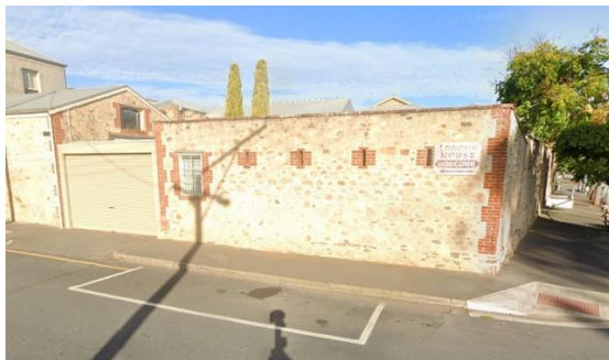
Stables at rear of London House in April 2023. Note the removal of render, and the addition of an enclosed garage with roller door.
