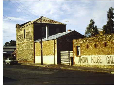
Similar perspective, taken 10 years later, showing the addition of painted signage on top of the cement render at the base of the stables.
