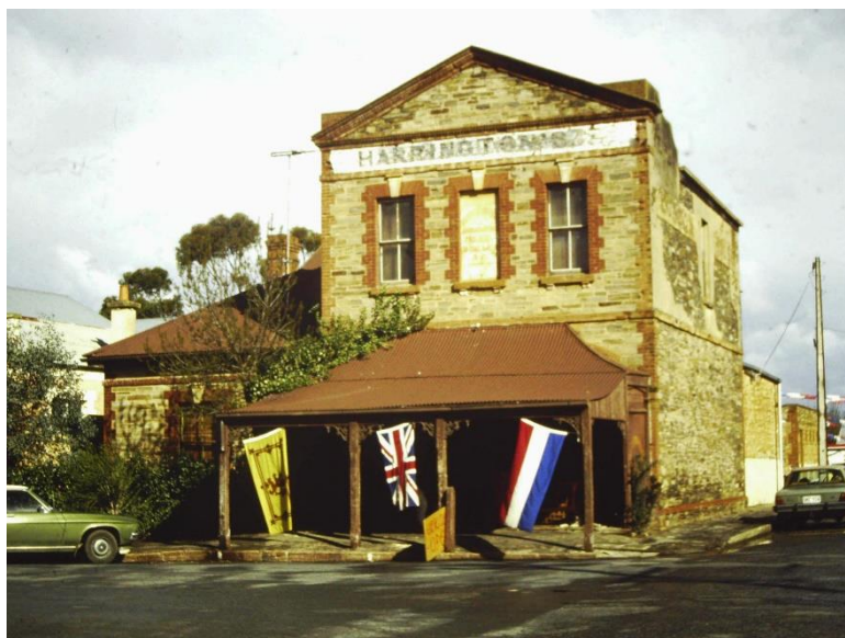
Photograph of London House 100 years later in 1981, prior to conservation.
