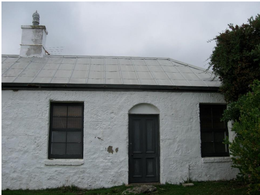
Portion of the eastern elevation towards the south, c.2011.
