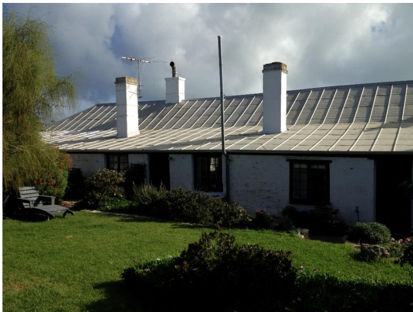
Western elevation showing backyard, c.2012.
