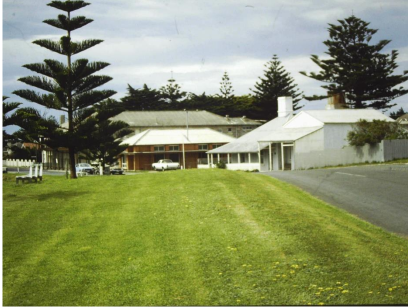
Western elevation of the former post office and telegraph station, c.1982.
