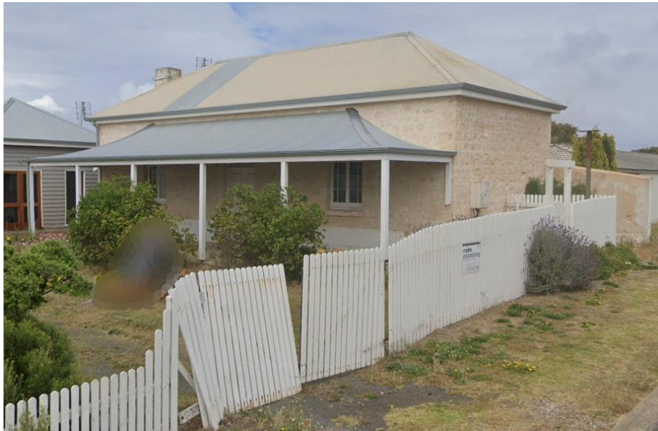
View of the front of the Courthouse in 2020, showing the removal of the paint and repointing of the walls, addition of the verandah and removal of the 'Police Station' sign.
