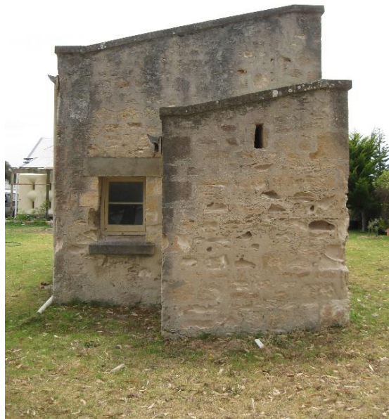
Southern elevation in 2012 showing removal of the render.
