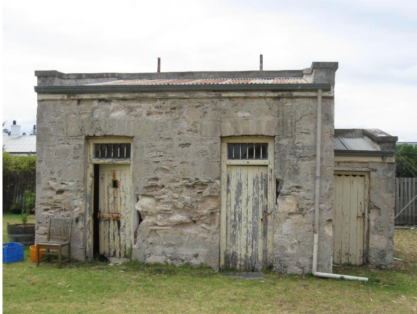
Front view of the Old Cells in 2012 showing the removal of the render.
