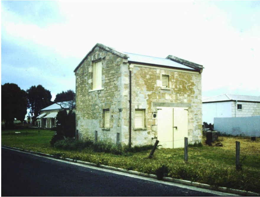
View of front and southern elevations of the Police Stables in 1981.
