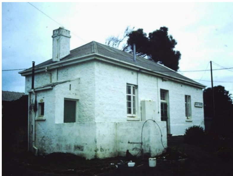
View of the Courthouse in c.1983 showing the lean-to to the southern elevation and the chimney. Source: DEW Files
