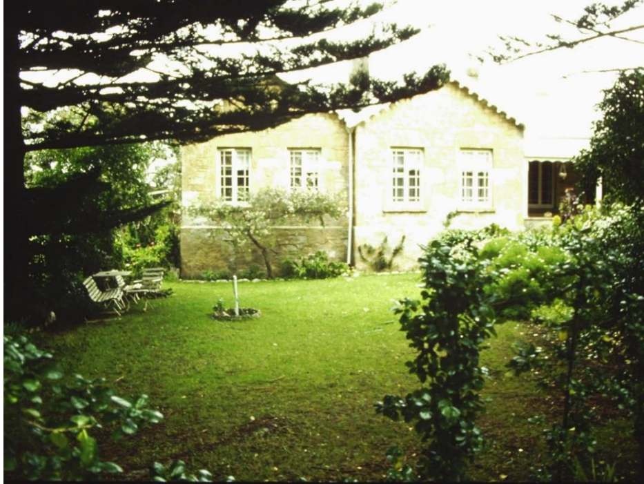
Two eastern wings adjacent to the front verandah, c.1983.
