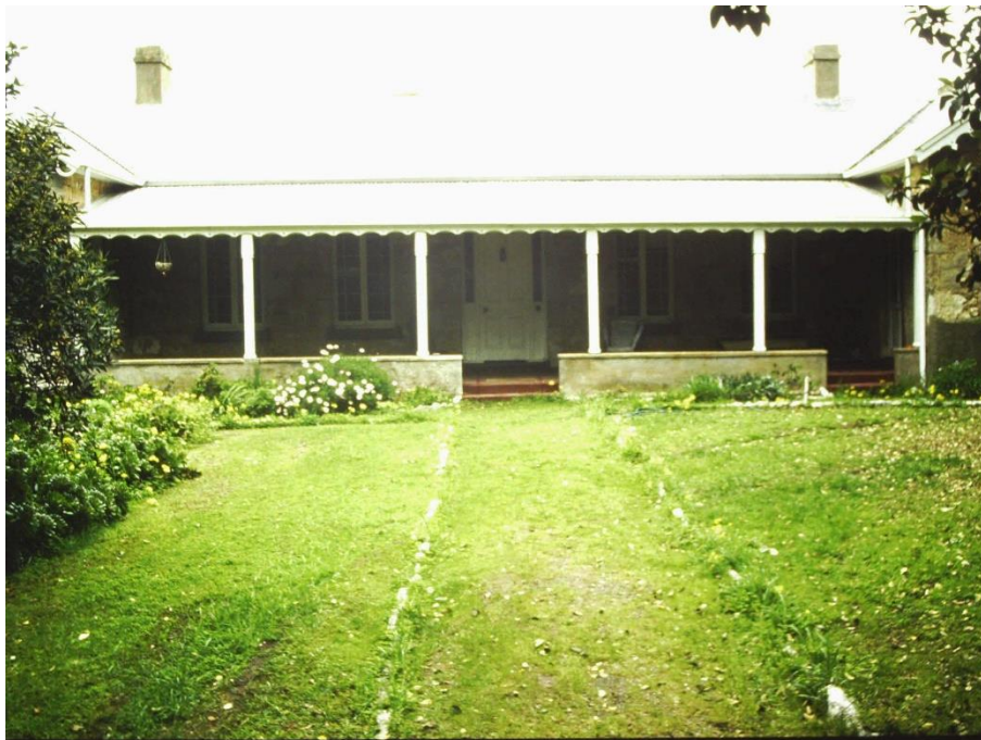
Part of the front elevation showing the verandah, c.1983.
