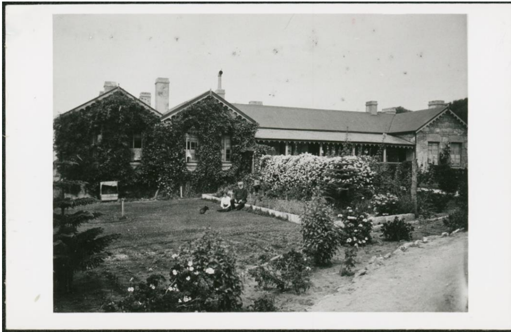
The front elevation showing extensive ivy coverage, c.1915.
