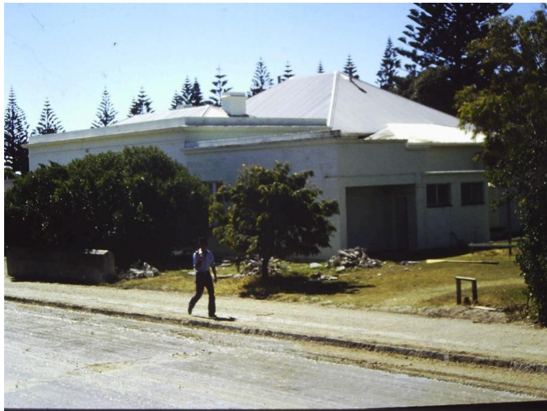
South-eastern corner of the Robe Institute with an extension to the east, c.1981
