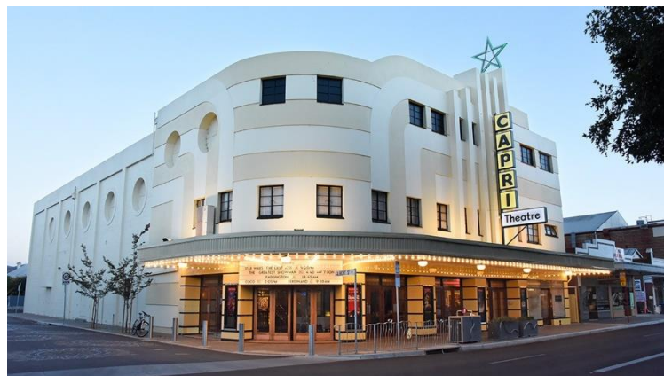
Capri Theatre (former New Goodwood Star Theatre) c.2018
