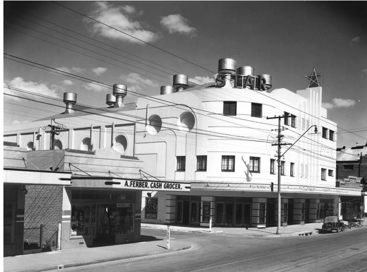
Capri Theatre (former New Goodwood Star Theatre) c.1941
