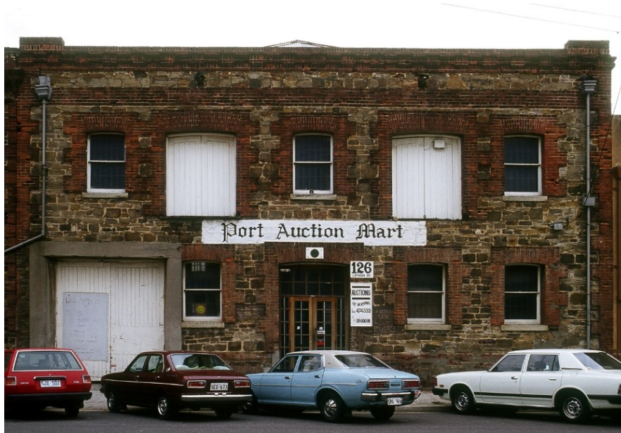
Former Elder's Bond and Free Stores, showing façade of 1863 store, c.1980.
