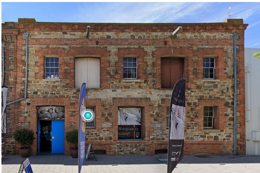
Former Elder's Bond and Free Stores, Lipson Street elevation of 1863 store after conversion to South Australian Maritime Museum display and interpretive centre, 2021
