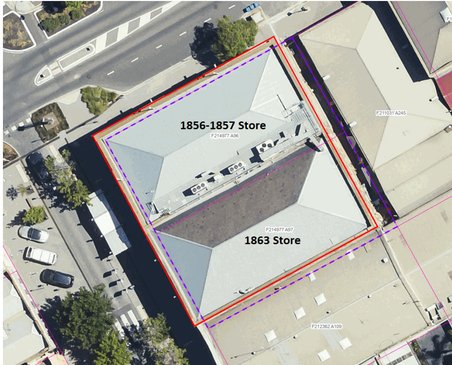
Former Elder's Bond and Free Stores, 126 Lipson Street, Port Adelaide SA 5015, CR 5598/388 A96, A97 FP 214977 Hundred of Port Adelaide, showing 1856-1857 and 1863 stores.*
