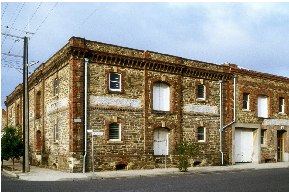
Former Elder's Bond and Free Stores, showing Divett and Lipson Street elevations of 1856-1857 store on left and part of Lipson Street elevation of 1863 store on right, c.1980.
