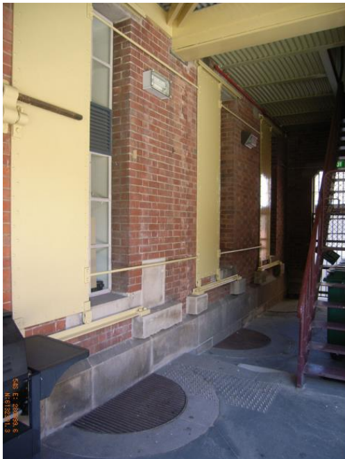
Steel window shutters and door security covers installed in the early twentieth century.
