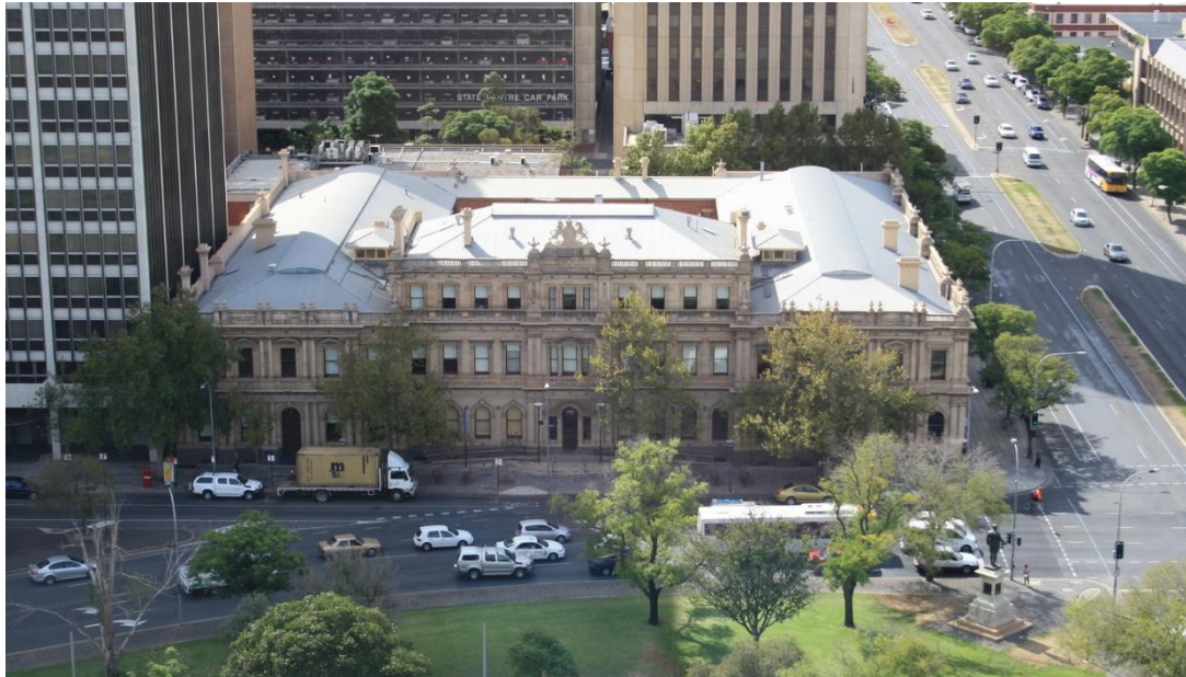
West elevation of the Torrens Building.
