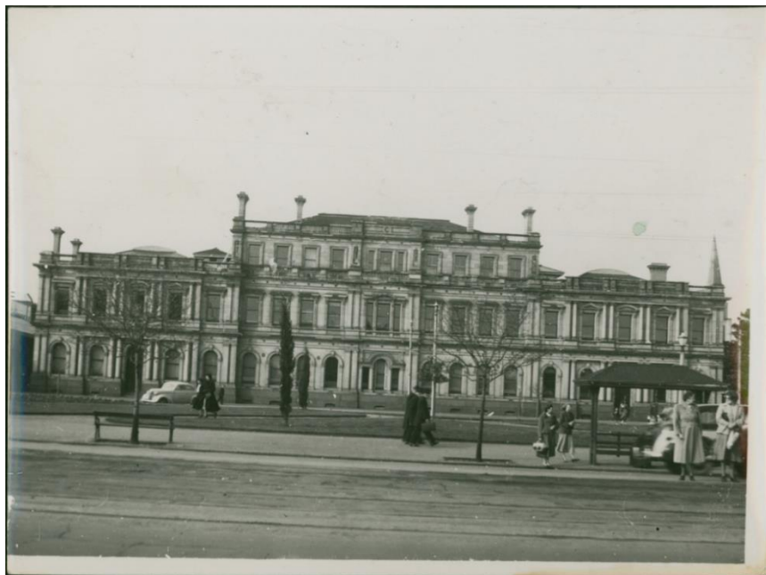
Western elevation of the Torrens Building in 1948. Note the missing coat-of-arms at the top of the centre bay.
