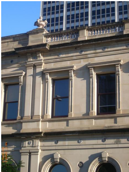
First floor windows to southern elevation.
