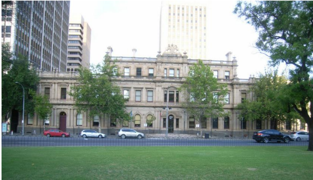
West elevation of the Torrens Building after conservation works in 2011. The British coat of arms has been added, and the centre windows on the ground floor have been modified to create a main entrance.
