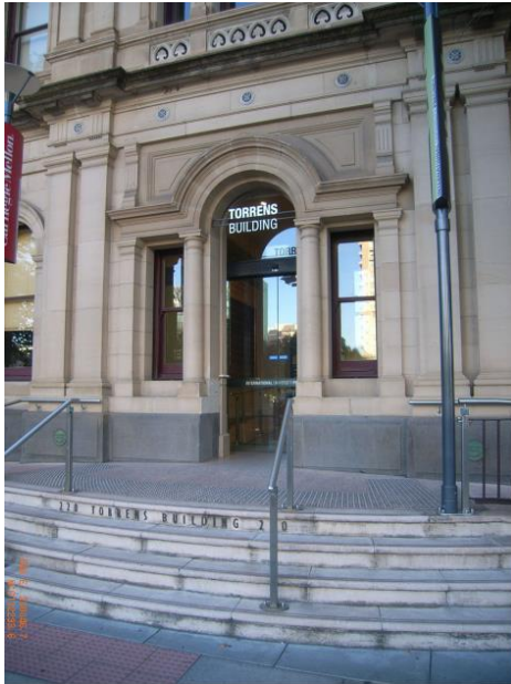
Central door opening to west elevation showing steps.
