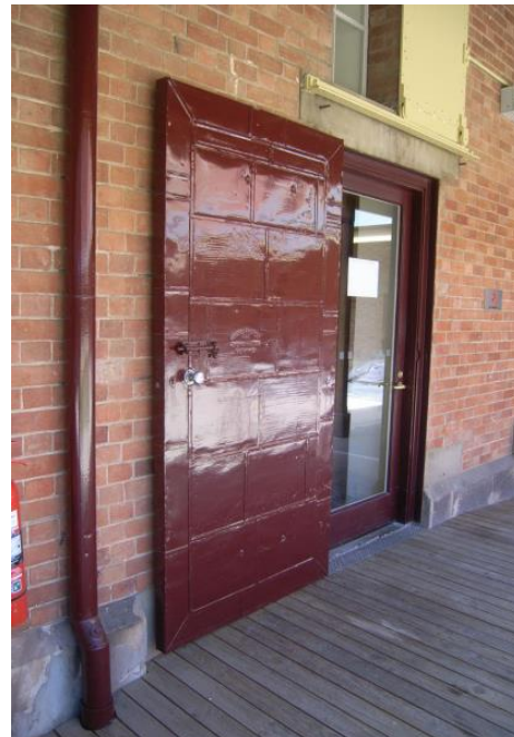
Steel window shutters and door security covers installed in the early twentieth century.
