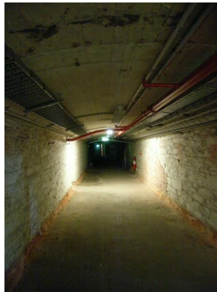
Central basement corridor to south wing looking east.
