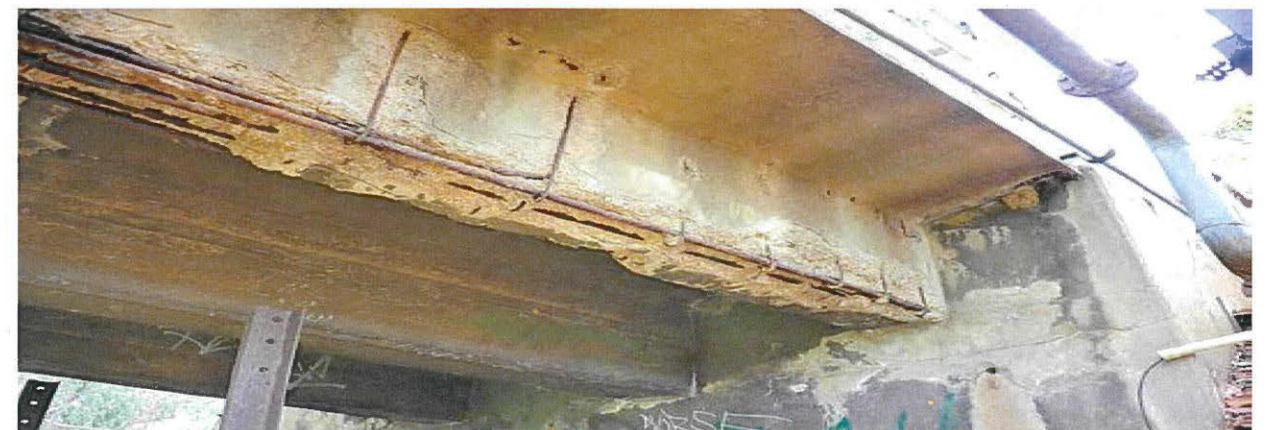
The outer beam on the eastern side in 2011 – this was the worst-affected beam and the one chosen for the trial repair in 2013 [Photo: John Woodside]
