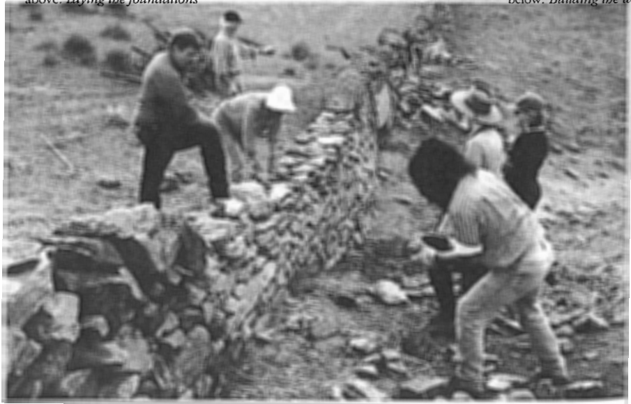
above: Laying the foundations
