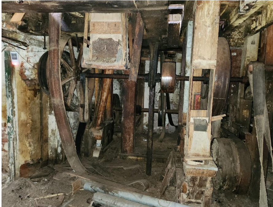
Milling equipment in situ in the basement of the flour mill.
