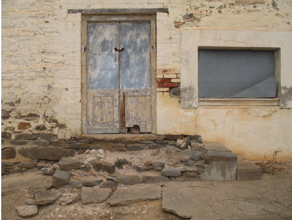
Entry door of the office from Commercial Road.
