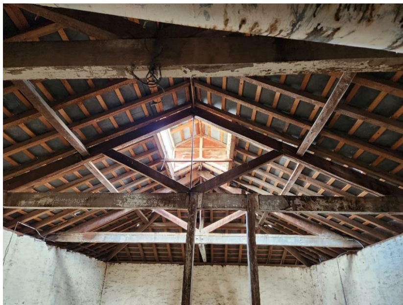
Interior view of roof lantern in the grain store.
