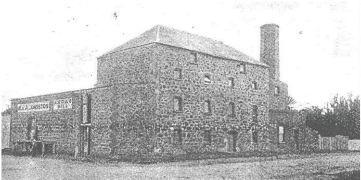
W. & A. Johnston's Mill c.1906. The steam engine boiler house and chimney stack to the right were later demolished to make room for a grain shed.
