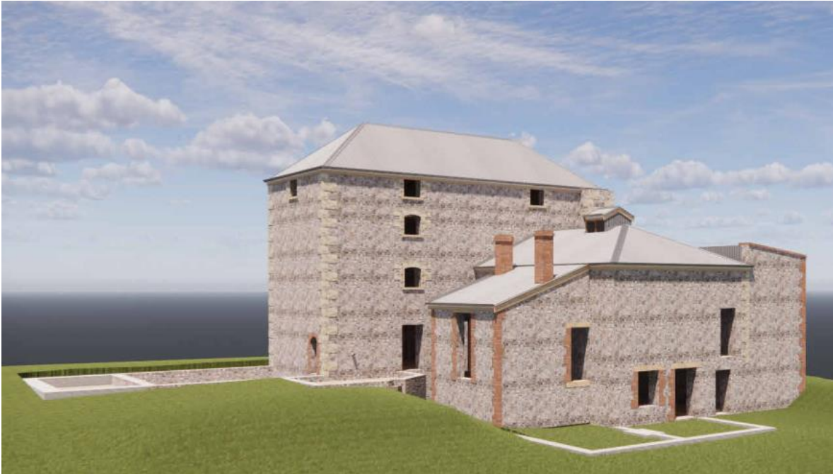
Rear of Angas Mill looking North. The steam engine and boiler room footings can be seen clearly on the buildings west and south elevations.
