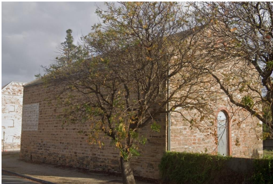
The west and north elevation of Colman's Store. The Angas Mill can be seen behind.
