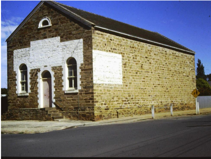
Colman's Store taken from the corner of Commercial Road and Mill Street in 1981. Note the painted quoins around the windows and doors, and the missing balustrade on the entry stairs.
