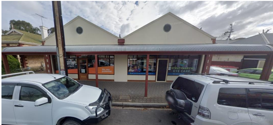
Shopfront of unit 3 facing Albyn Terrace.
