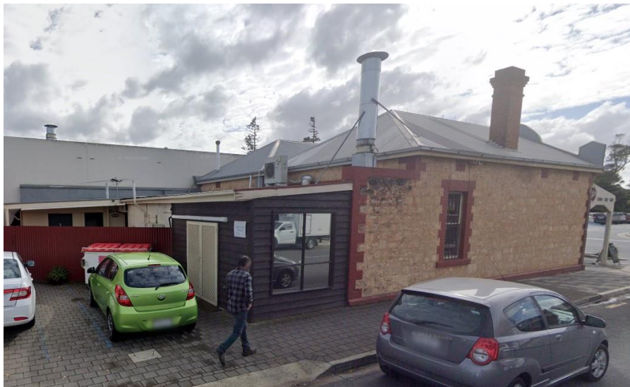
Southern elevation of Shops along Albyn Terrace showing the L-shaped lean-to extension.
