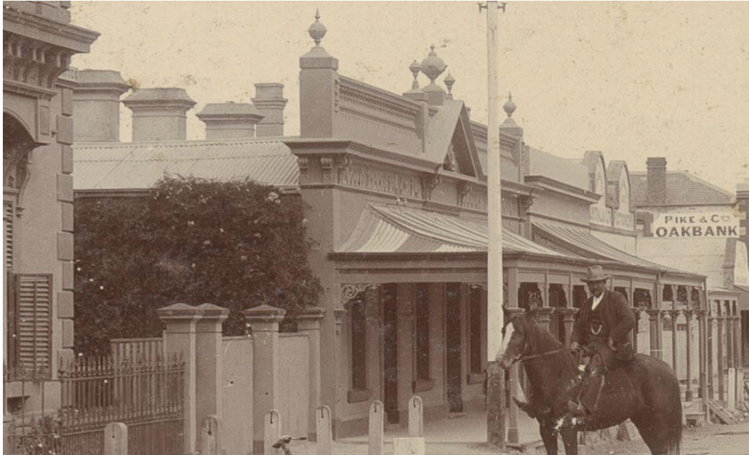
Close-up showing the updated façade. Signage for Bagot, Shakes and Lewis is painted on the building new entablature.
