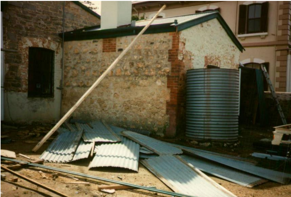
Rear of 4-6 Albyn Terrace during conservation works in the late 1990s.
