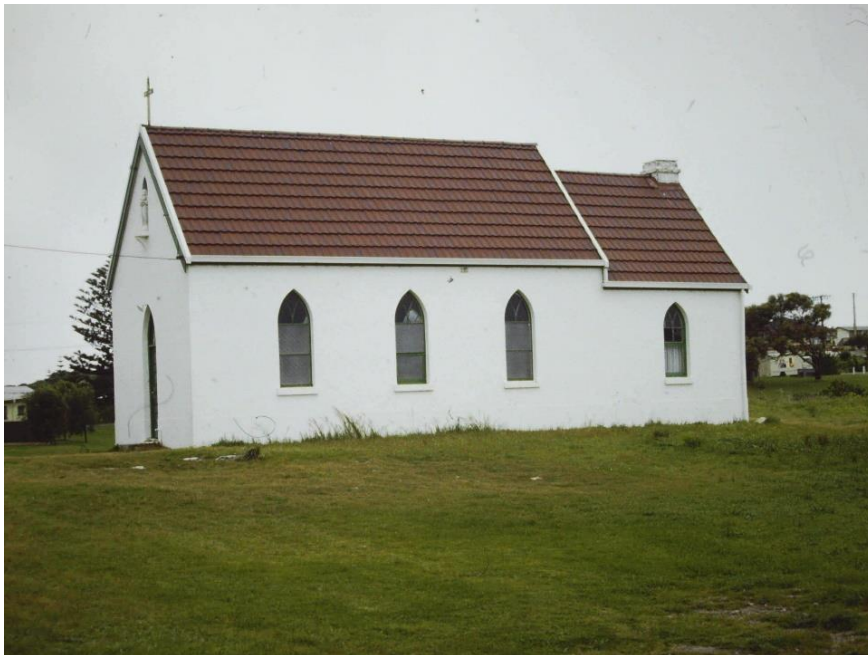
North-facing elevation of the chapel with lean-to to the rear, 1980.
