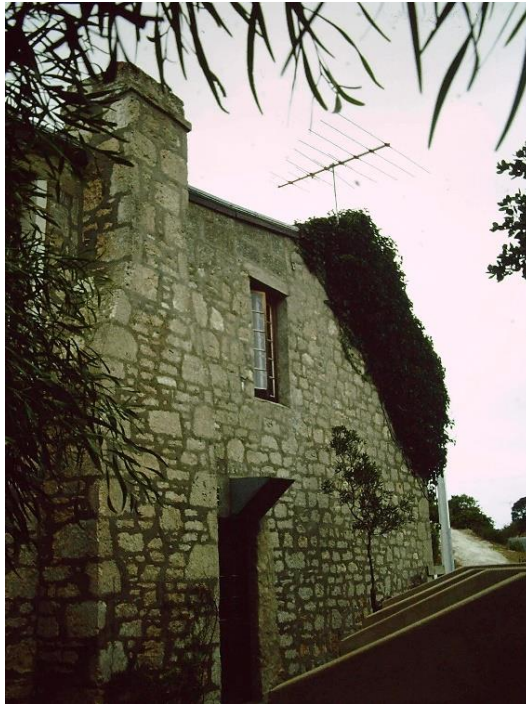
Western elevation, c.1982.
