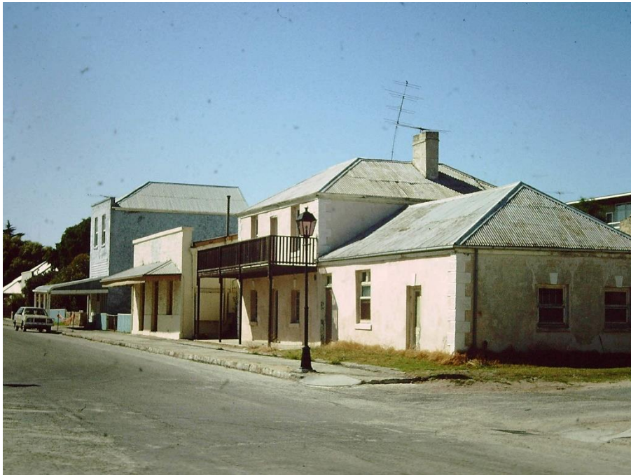
View of the Former Criterion Hotel showing the western elevation, c.1983.
