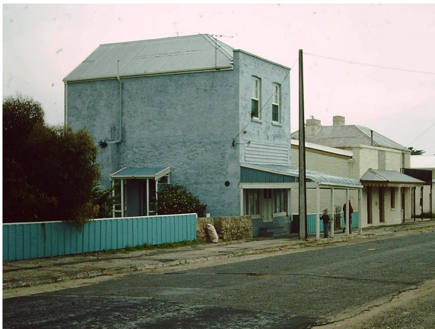
Eastern elevation of Davison's Shop, showing Former George Lord's Horseshoe Forge (LHP) and the Criterion Hotel (SHP 12539) to its right, c.1981.
