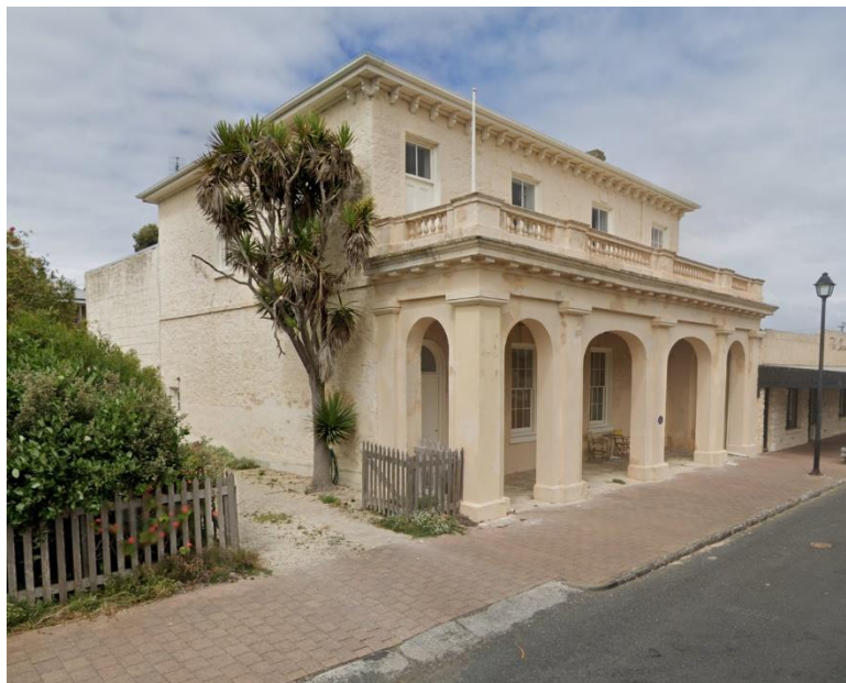
Bank House, November 2020
